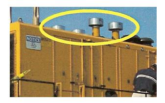
Stainless steel rotor Cast aluminum body Polished aluminum hood Dual sealed ball bearings
